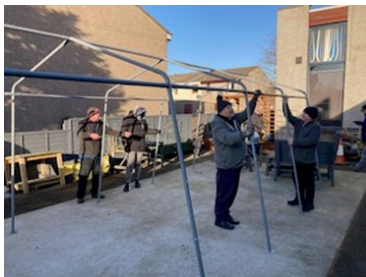
Members assembling temporary outside workshop.
