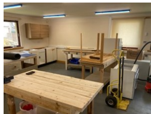
Workshop during refitting
