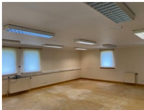
Main workshop before refitting
